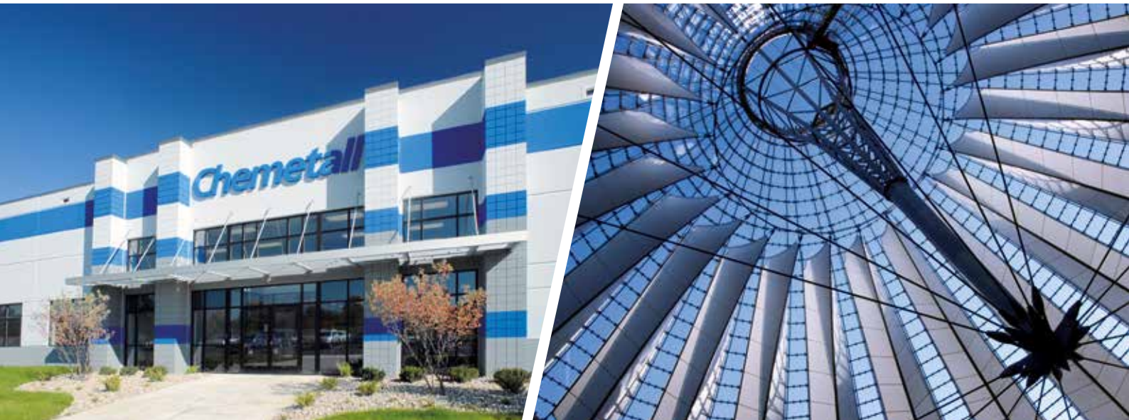
Largest surface treatment facility in the world (Jackson, MI, USA)
